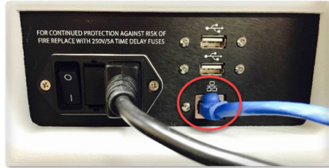
Figure 4. Ethernet port with wired network connection cable
