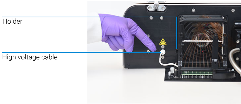
Figure 54 Instrument top compartment – high voltage supply cable
